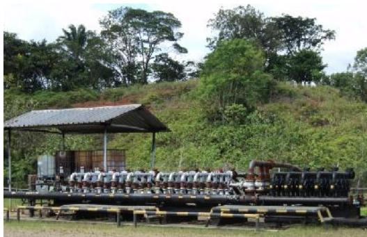
Fig. III. 6. Manifolds
