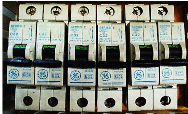
Figura 41. Disyuntores General Electric C-32
