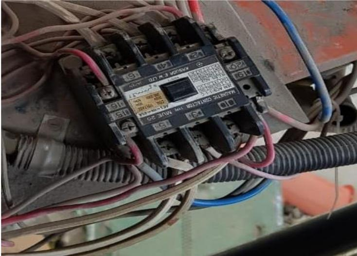
**Figura 39-3.-**contactor #1 del motor-reductor carro transversal.
