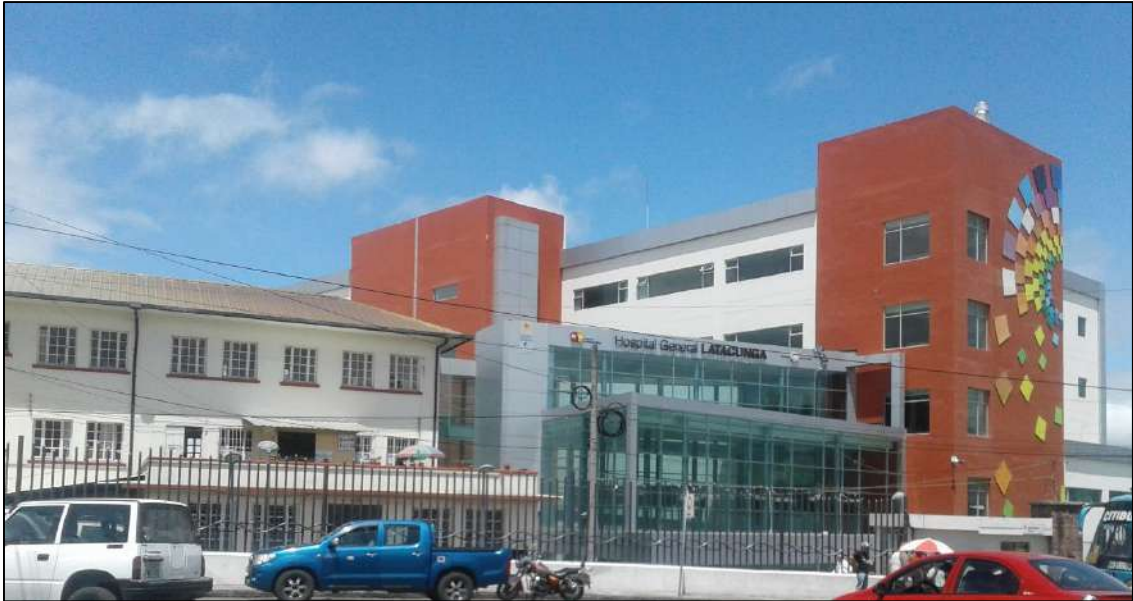
Figura 1-1: Hospital General de Latacunga
